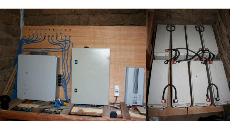
Meter and communication box (previous page), electrical protection and PCU (above) and batteries bank (above right)
